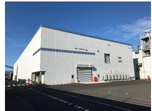
Tsuruga Films Plant Coater Building
